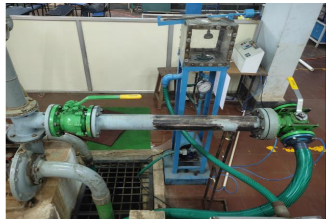
Fig 3.1.3 Pipe connected to 2 & 3 way Valve
